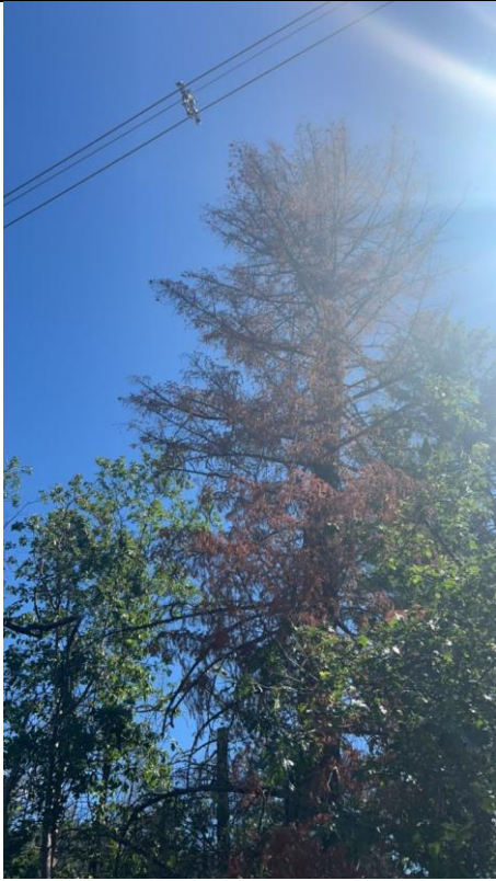
Photo 3: Photo of the dying pine tree located approximately 15 feet northeast of the primary conductors.
