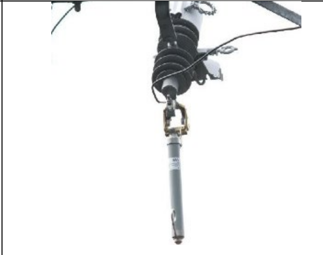
IA1mg2: Exempt fuse in the open position in its cutout (close view).
