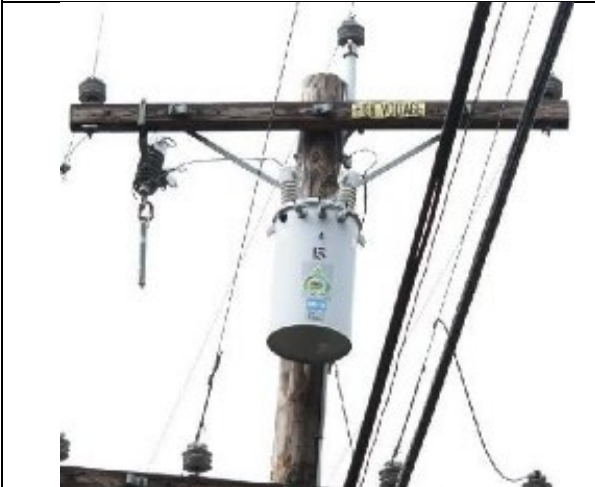
IA1mg1: Exempt fuse in the open position in its cutout.
