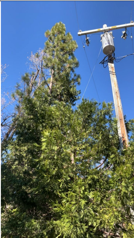
IA1Img3: Vegetation in contact with the pole and guy wire above the insulator
