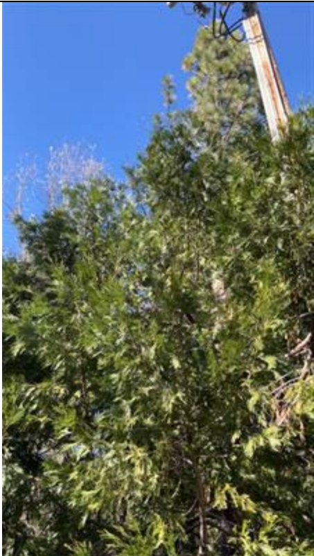
IA1Img7: Vegetation in contact with the pole and guy wire
