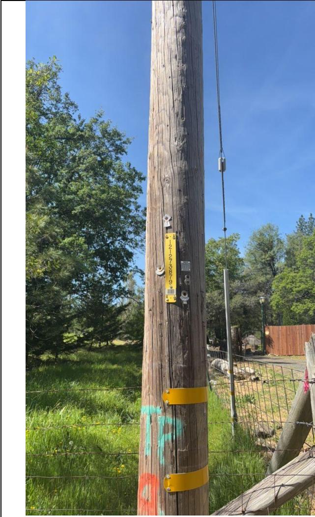
Photo 1: Photo of pole ID 121273879
