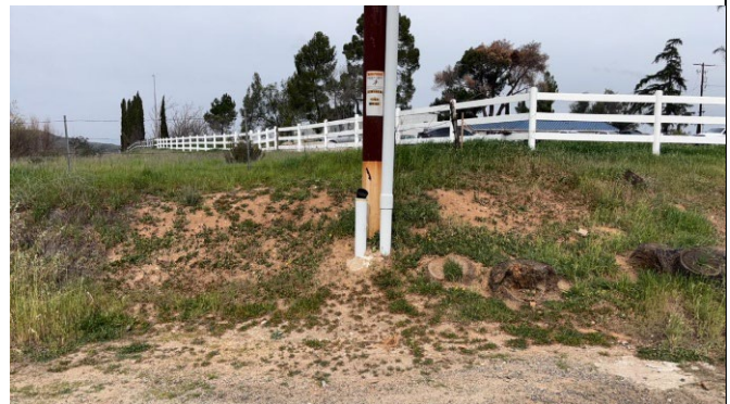
Photo 4: Overview of the pole and regrowth of vegetation within the 10-foot radius of the pole, taken during the inspection on February 10, 2026
