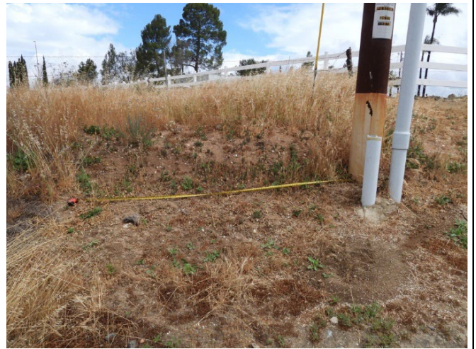
Photo 6: View of annual vegetation and desiccated stumps within the 10-foot radius of the pole, taken during the inspection on February 10, 2026.
