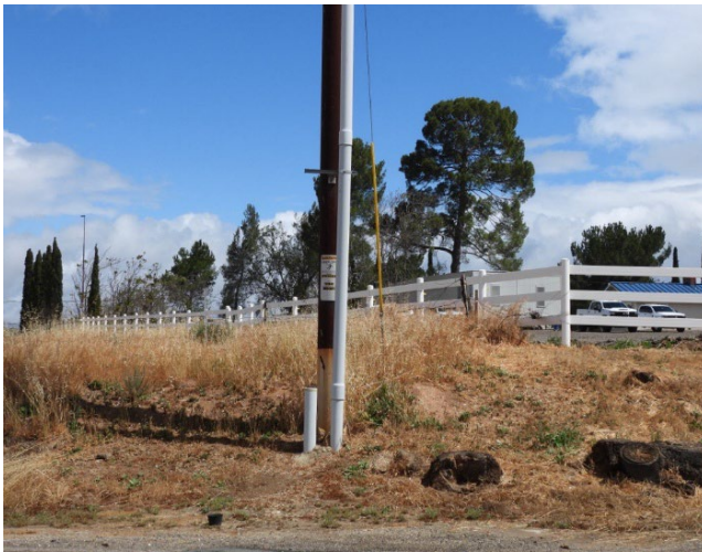
Photo 7: Overview of dry fuel source around pole ID P610587, taken during the inspection on April 13, 2026.
