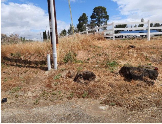
Photo 9: Additional photo depicting the 10-foot radius from pole ID P610587, taken during the inspection on April 13, 2026.
