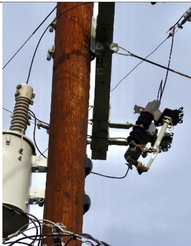
IA1Img2: Non-exempt expulsion fuse in use example 2.
