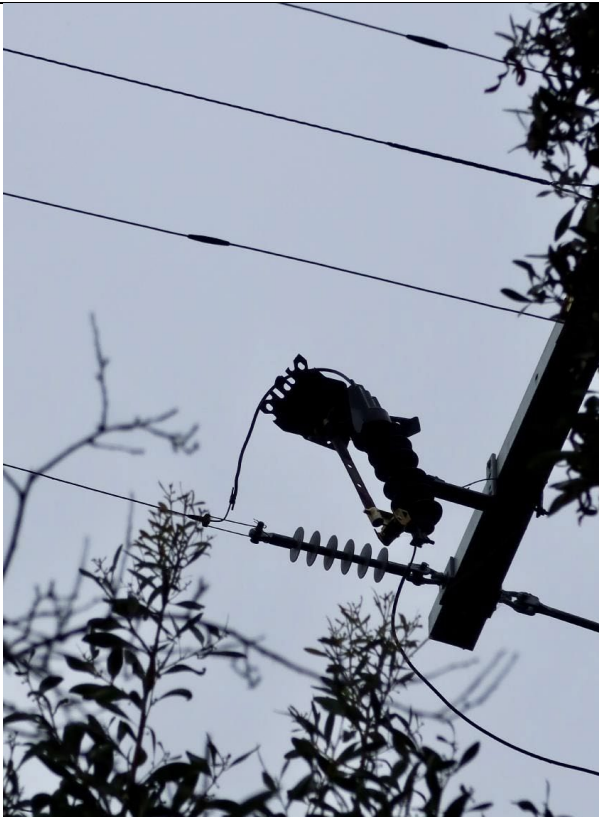
IA1Img3: Solid blade disconnect one.
