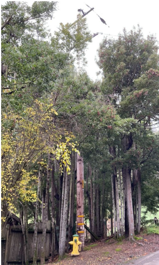
G1mg1: Overall Structure without 10 feet of vegetation clearance.
