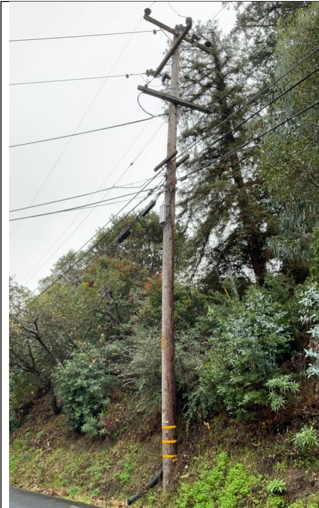
G1mg1: Overall Structure.
