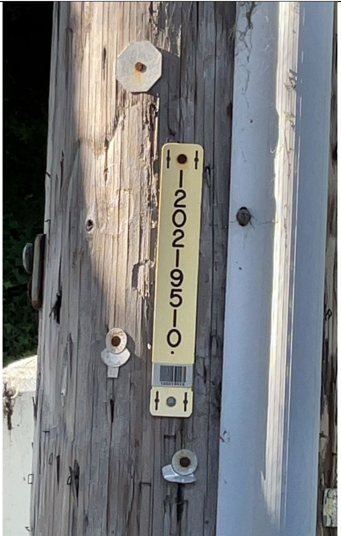
Gimg2: Structure ID.
