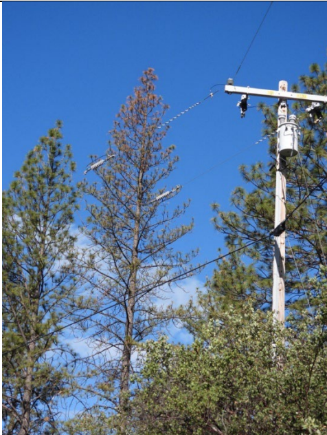
Photo 3: Photo of the dying Jeffrey pine tree near the conductor.
