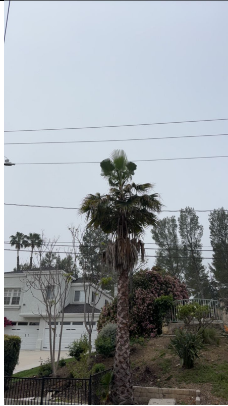
Photo 4: Additional photo of the Mexican palm tree encroaching within the four-foot minimum clearance distance from the primary conductor. Photo taken south of the tree looking west.
