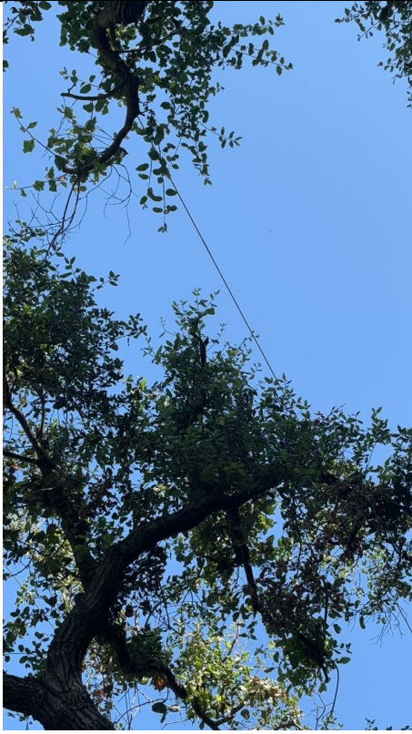
Photo 3: Close-up photo of the same oak tree encroaching within the four-foot minimum clearance distance from the primary conductor.
