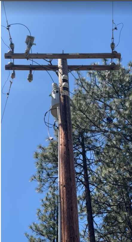
Data Inaccuracy Img3-1: East view of the pole showing no covered conductor on the east portion of the pole.
