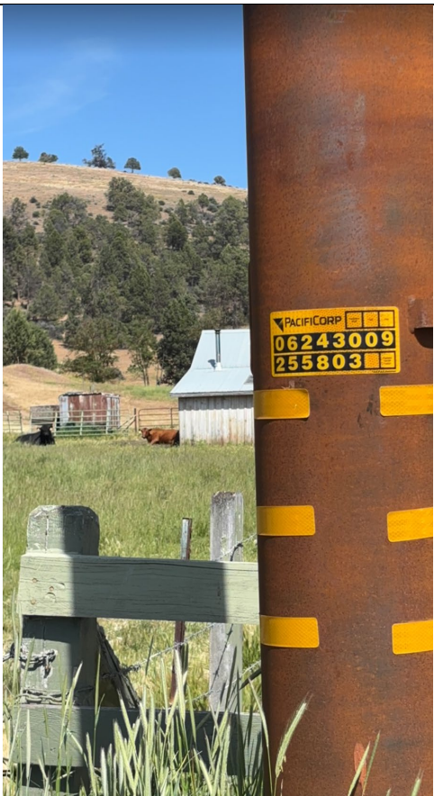
Data Inaccuracy Img10-2: Structure ID - 062430090255803
