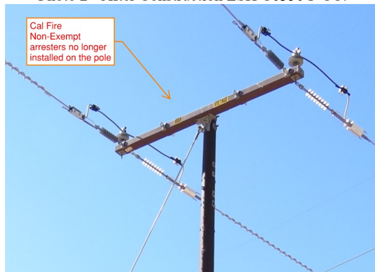
Photo 2 - After Construction ESH C0350 P CC:
